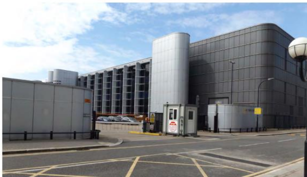
View A - From South East
